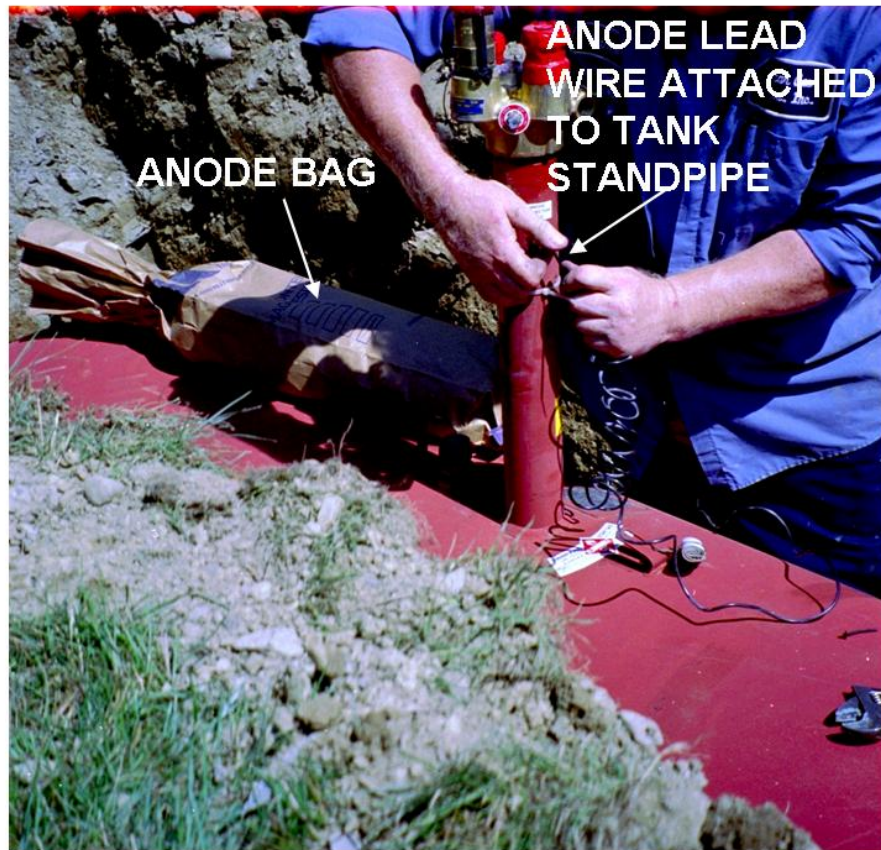
Figure 2. Installation of Cathodic Protection System on Underground Propane Tank
